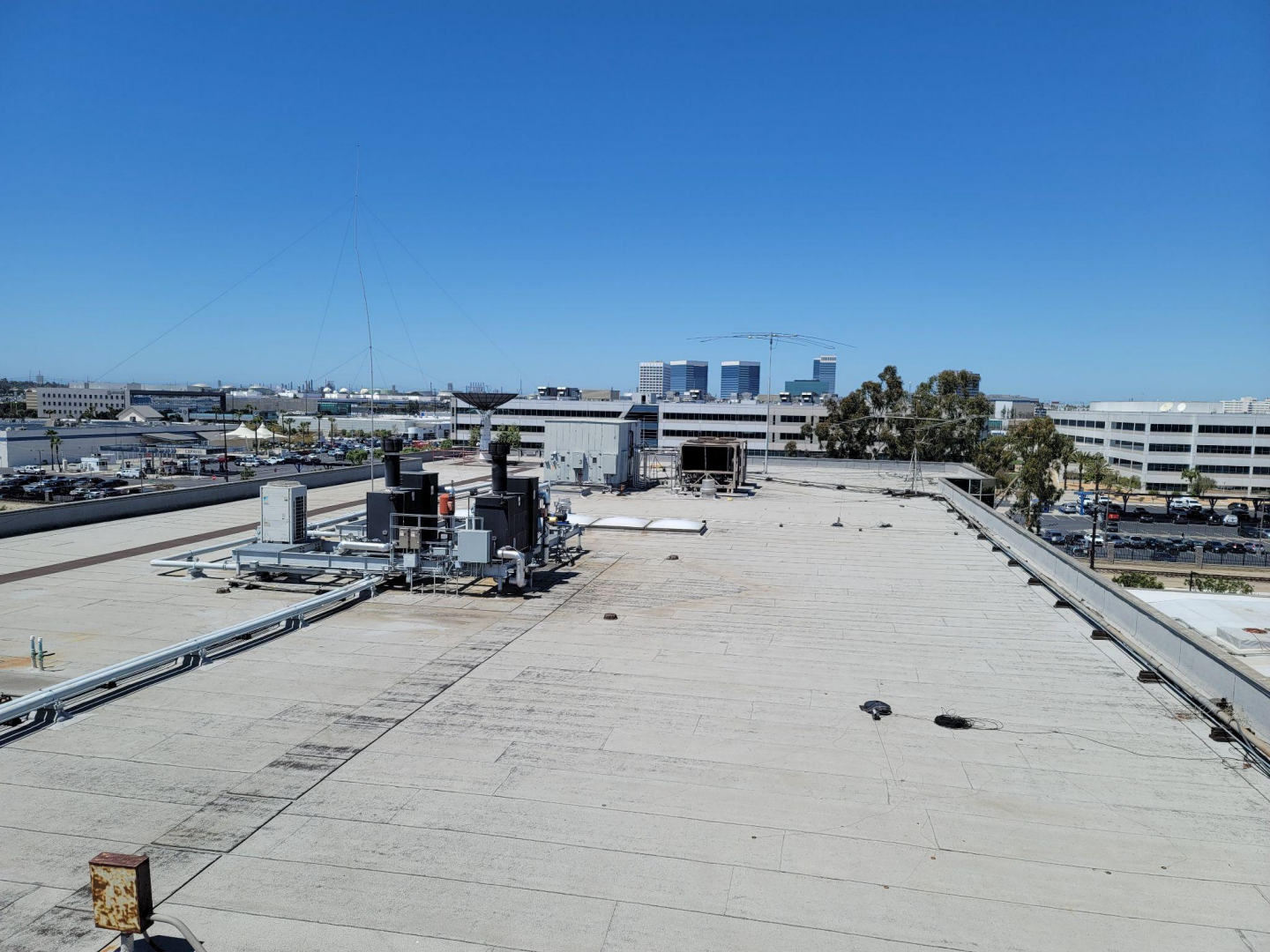
View from top of penthouse
